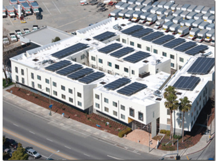
Two 3672 systems provide water for the entire 180 unit building
